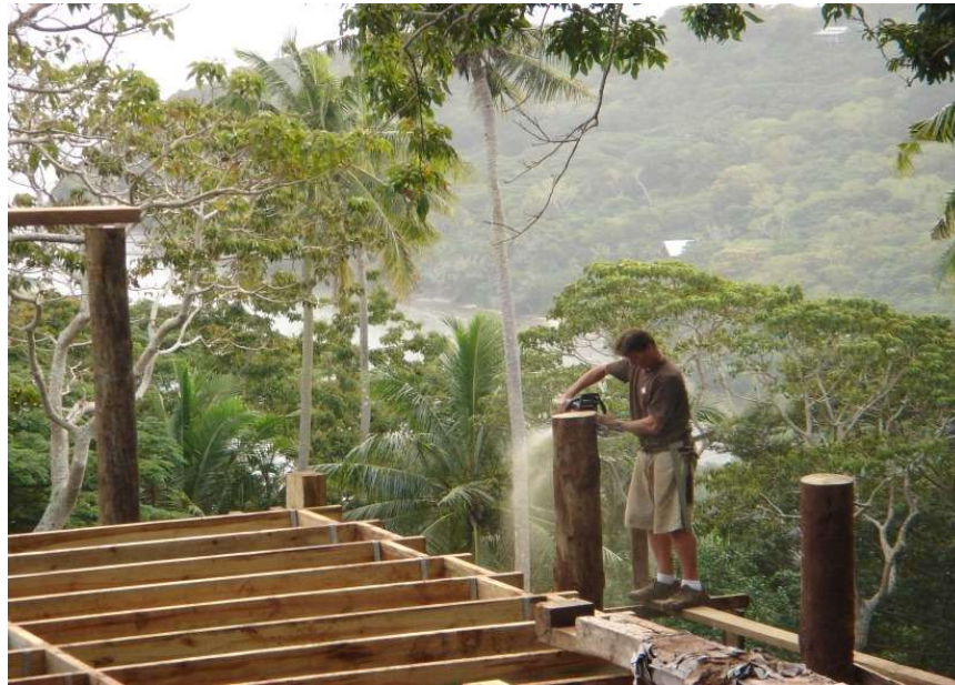
Framing a deck with the rainforest and bay behind
